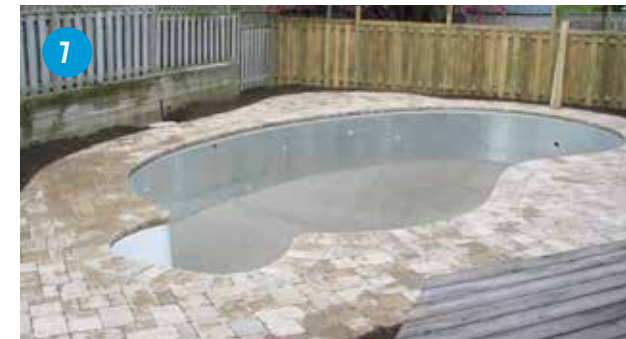
7 Hand Troweled Concrete Bottom
