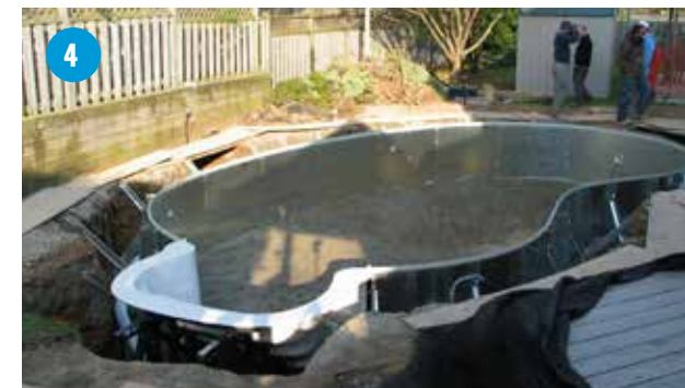
4 Plumbing Run And Trenched Underground
