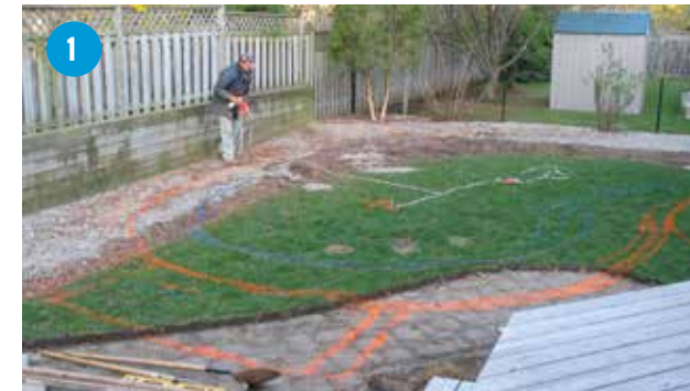
1 Pool Shape Staked Out For Excavation
