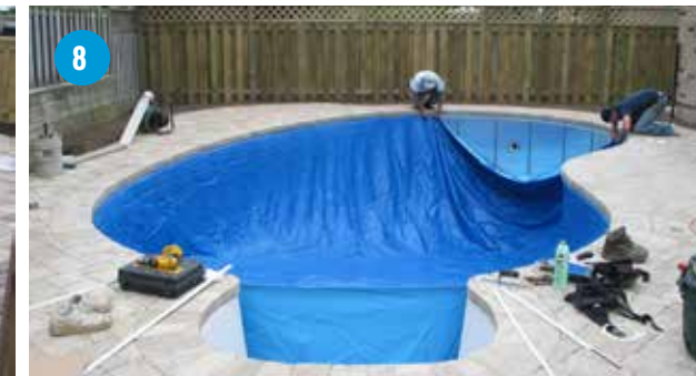
8 Liner Installed
