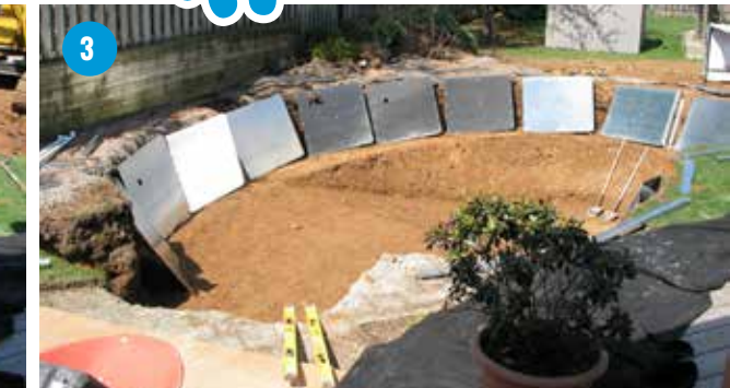
3 Walls Placed And Levelled
